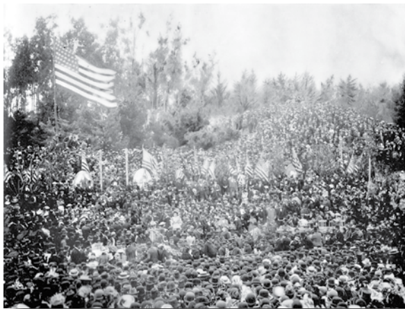
I. W. Taber's 1893 photograph of the official ground-breaking ceremony.
